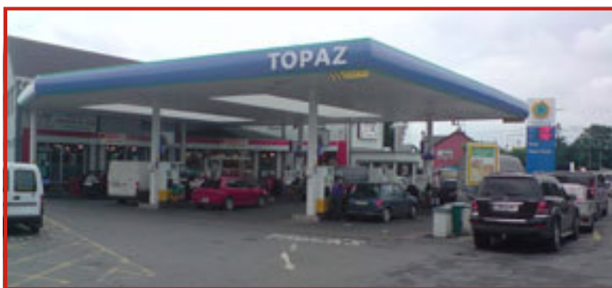
Getting Connected: Corrib Oil's SPAR Express store in Tuam, Co. Galway
